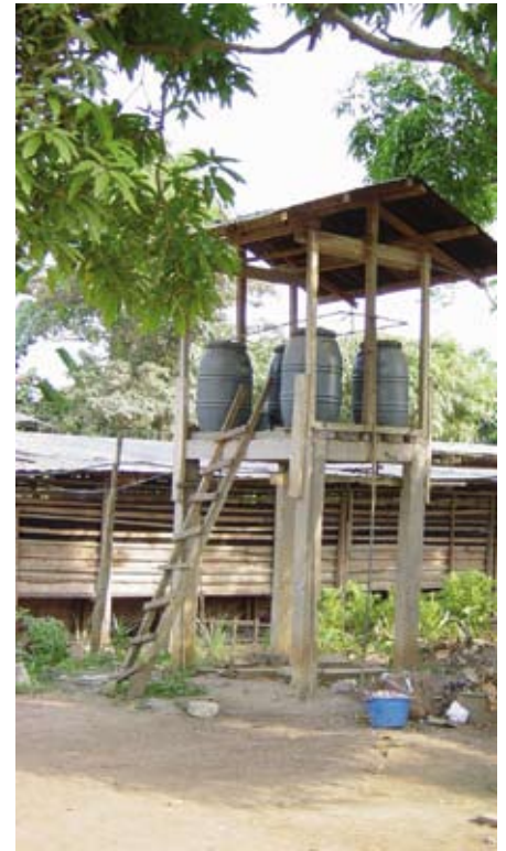
The tanks should be light in colour, shaded and filled up to 80% capacity to keep the water cool.
