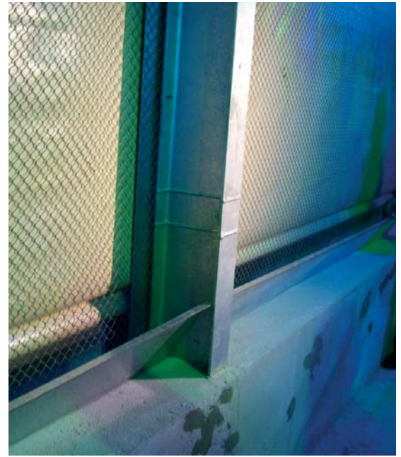
Roll Seal curtains are insulated, double covered, light and air tight.
