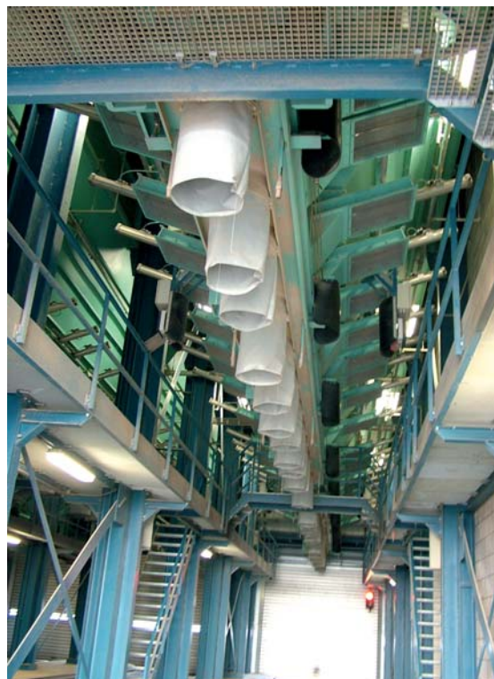
One of the five load-out lanes with the contrasets on top that march the compartments in the bulk truck.
