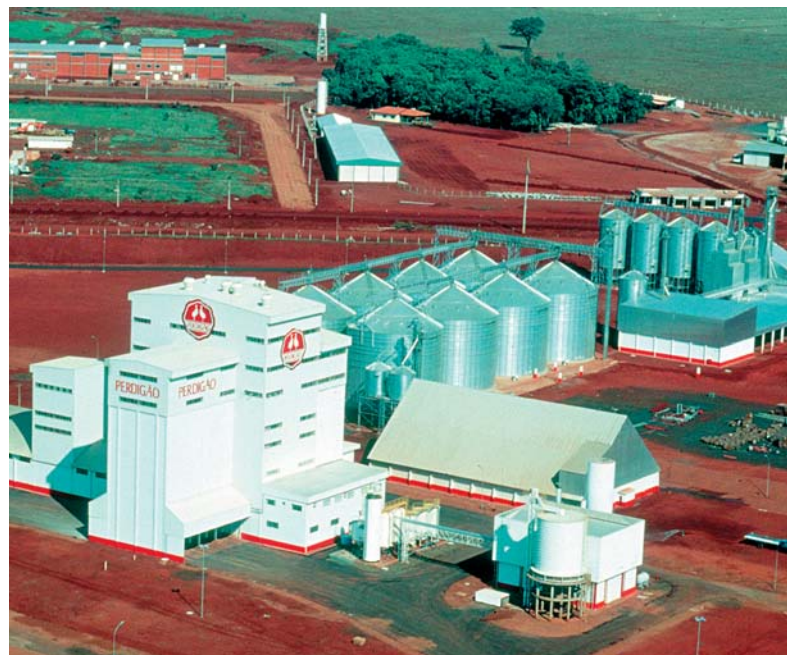
Perdigão's complete feed plant with a capacity of 120 t/h is part of a food complex with a total investment of US$ 250 million. Located in the background is the cereal intake with drying facility and storage in large silos. On the right hand side the boiler house can be seen and behind it the flat storage facility for soy extraction meals. In the centre is the feed production plant with bulk load-out tower. On the left a premix plant is incorporated with a capacity of 5 t/h. (Photos: Bühler)
